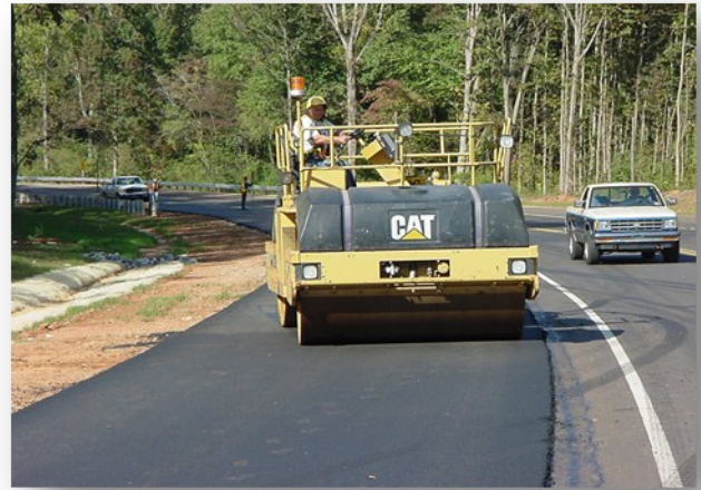
Compaction of an asphalt overlay.
