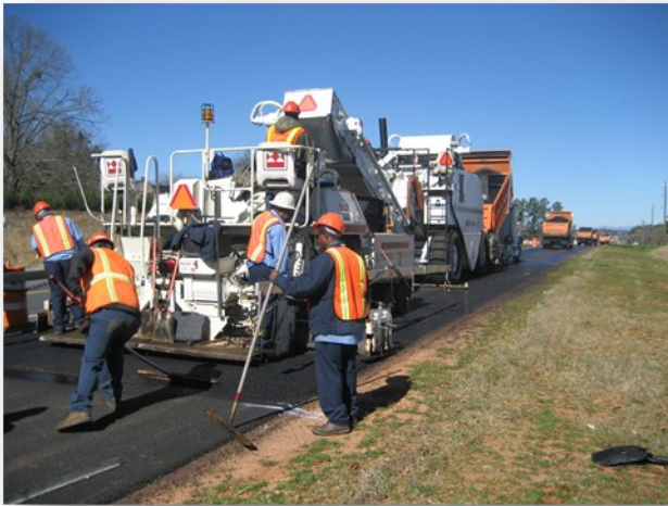
Placement of an asphalt surface course.
