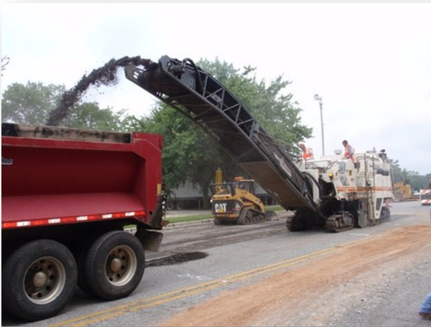
Removal of a controlled thickness of asphalt pavement using a milling machine.
