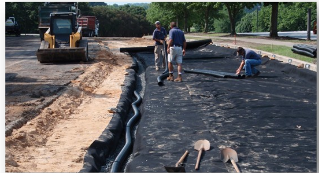
Installation of a pavement underdrain.
