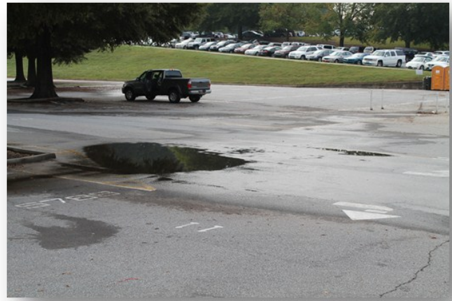
"Bird bath" due to inadequate pavement slope.
