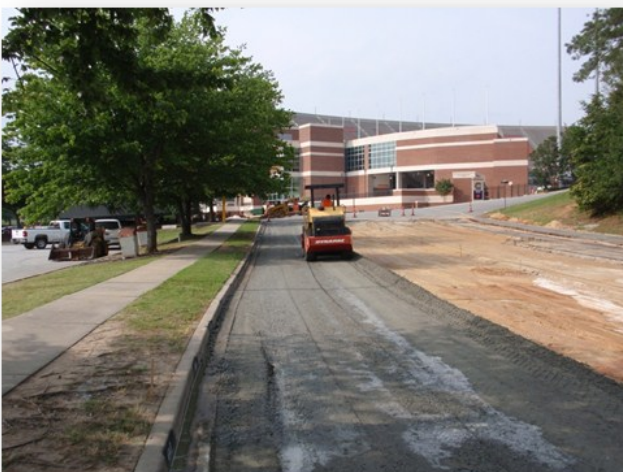
Preparation of subgrade and aggregate base course.
