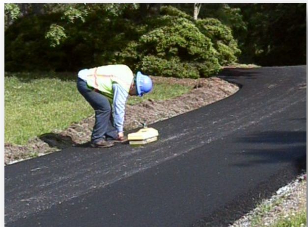
Measuring pavement density with a nuclear density gauge.
