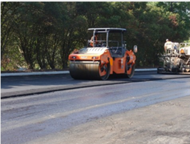
Initial breakdown compaction of an asphalt surface course.
